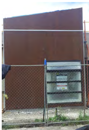
0 MONTHS: Recently built, this shows the beginning colour of Weathertex Natural boards.
